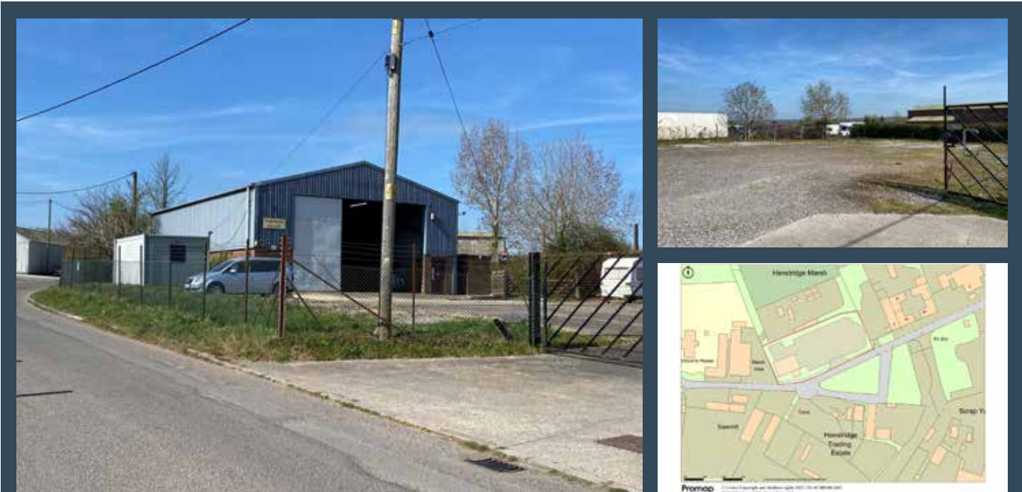
A lofty workshop with large and level fenced outside space
