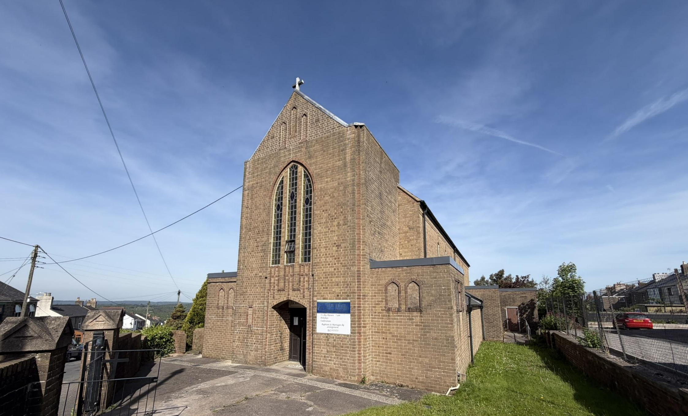
Former Our Lady of Victories Catholic Church Flaxley St, Cinderford GL14 2DJ
