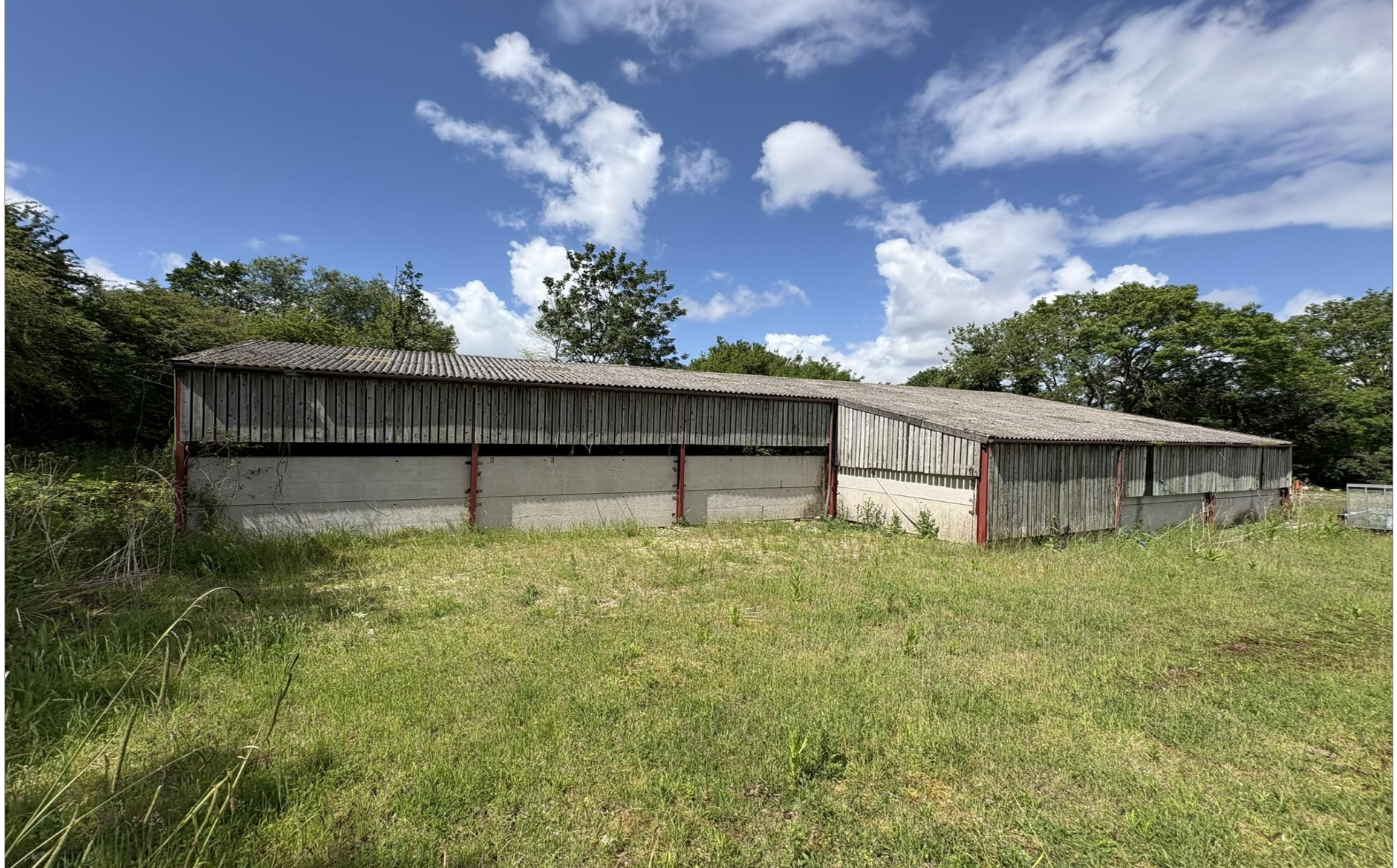
Barn at Church Farm Cottage Queen Charlton, Near Bristol, BS31 2SQ
